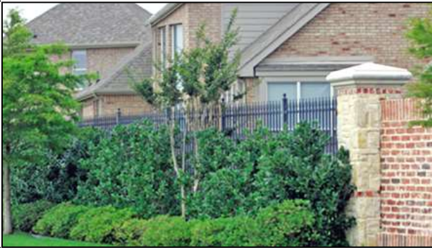
Type 2: Wrought Iron with Masonry Columns
