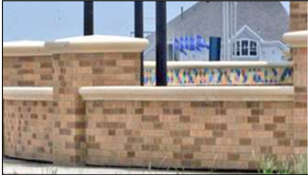
Type 1: Masonry Construction
